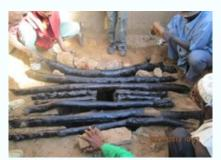
**3.** A wooden slab is prepared and coated with engine oil to protect the wood from termites.
