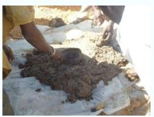
**5.** Plastic material is used to cover the top and reduce water leakage.
