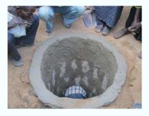
**3.** The inner walls of the pit - from top to bottom - are stabilized with bricks.
