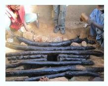
**4.** The wood of the slab is coated with engine oil to protect it from termites and leaking water.
