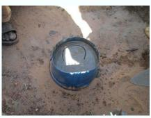
**8.** The cover is made from a mixture of cement and sand in a hand crafted mold.
