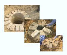
**7.** For the model without wood, bricks are stacked upward giving a conical shape at the top.
