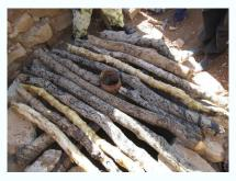
**3.** The wood is coated with engine oil to resist termite attacks.
